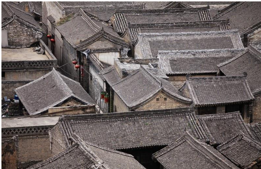
Figure 3. 1 Traditional 'Guanzhong' Courtyards
